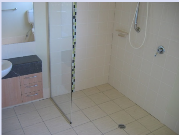
Figure 7.1 Image of a step-free and hobless shower with glazed screen, no door
