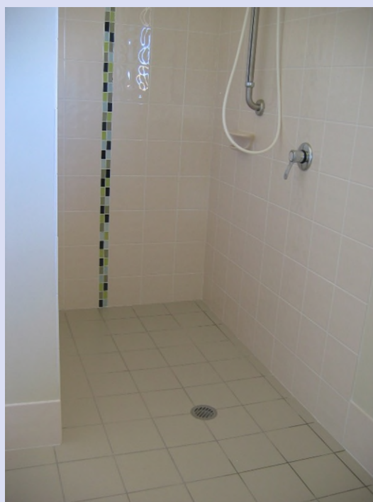
Figure 7.2 Image of a step-free and hobless shower with no screen
