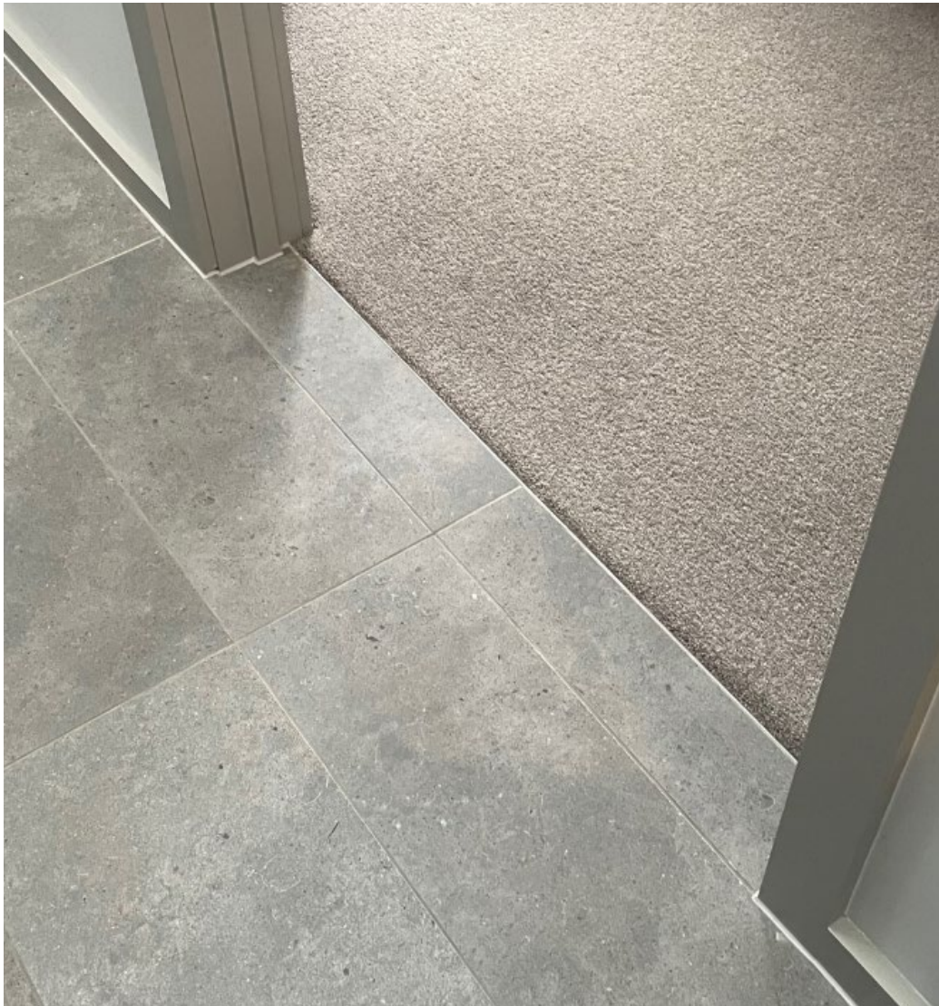
Figure 5.3 Example of a level threshold through the doorway
