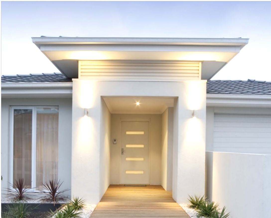
Figure 4.8 Front porch area with roof cover over landing area
