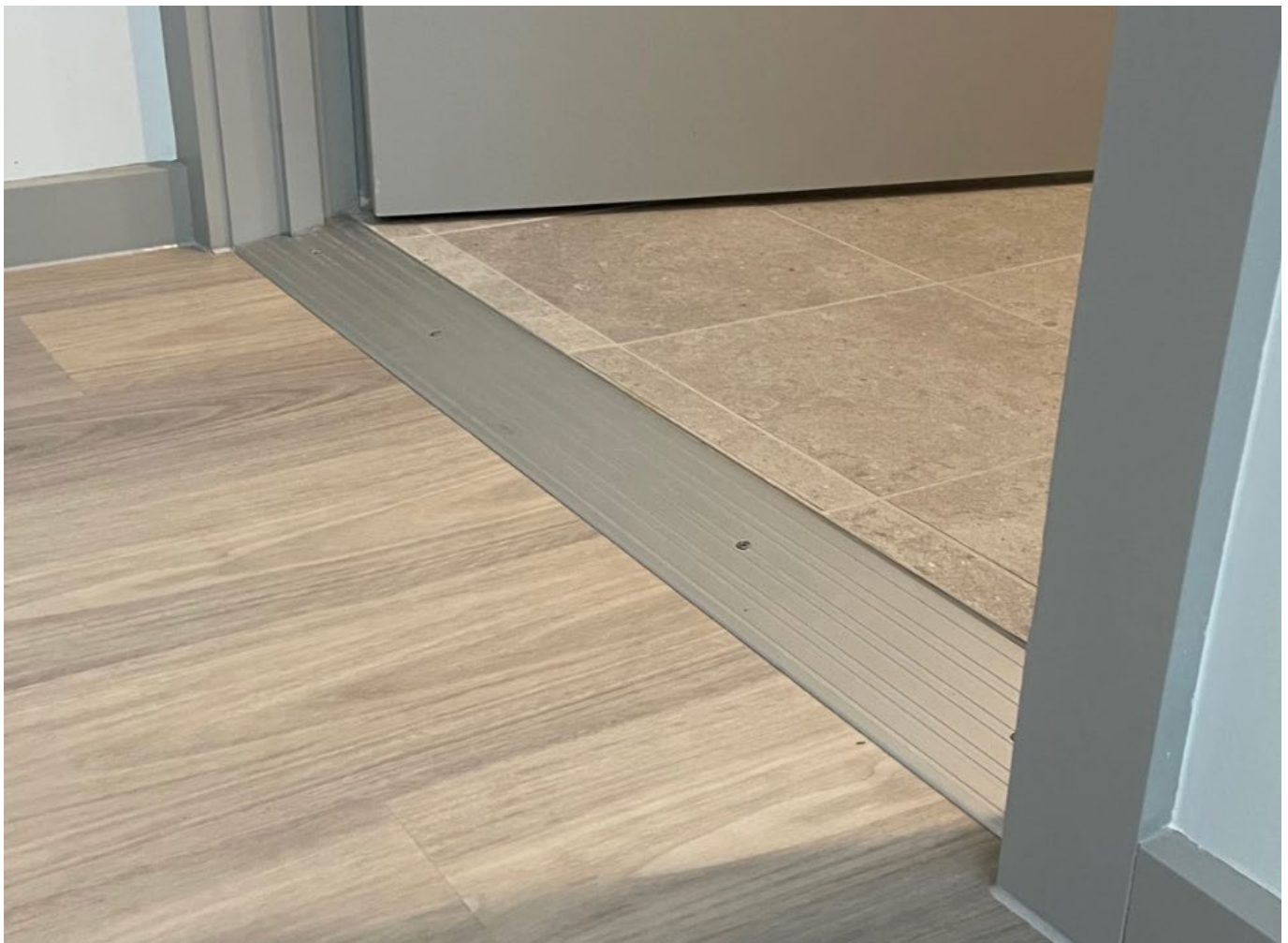
Figure 5.2 Example of a ramped threshold within a door jamb
